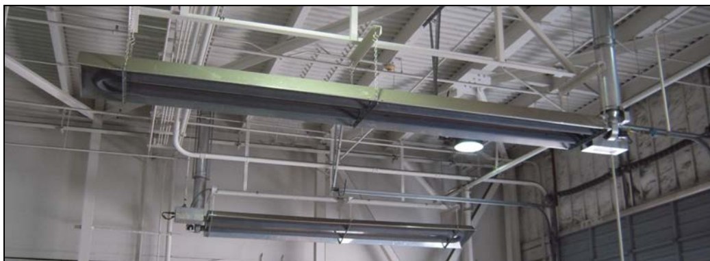
Figure 8: Gas-fired infrared tube-type heater. Photo courtesy of Gladstein, Neandross & Associates, NREL
