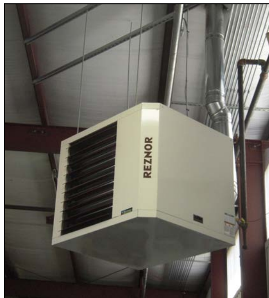
Figure 11: Gas-fired fan heater. Photo courtesy of Gladstein, Neandross & Associates, NREL
