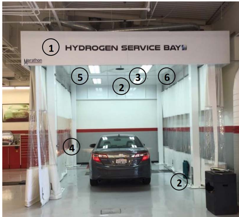
Figure 19: Hydrogen Service Bay, Annotation descriptions below. MarathonSprayBooths.com
