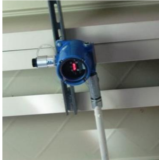
Figure 4: A ceiling-mounted combustible gas detection head. Photo courtesy of Gladstein, Neandross & Associates, NREL
