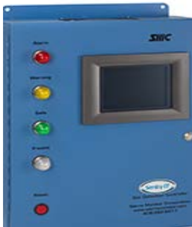
Figure 7: A combustible gas detection system control panel. Photo courtesy of Gladstein, Neandross & Associates, NREL
