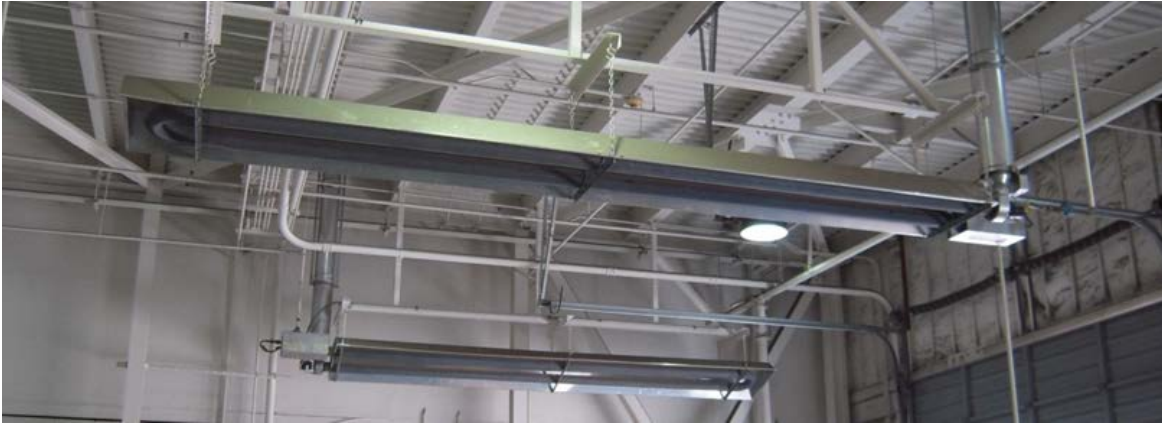
Figure 19: Gas-fired infrared tube-type heater. Photo courtesy of Gladstein, Neandross & Associates, NREL
