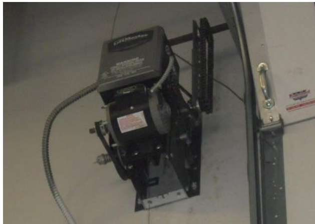
Figure 27: A typical electric door motor. Photo courtesy of Gladstein, Neandross & Associates, NREL
