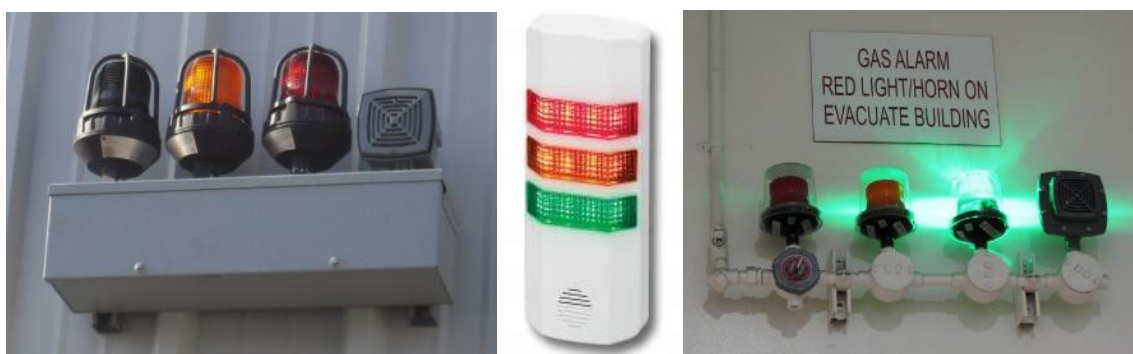
Figure 6: Examples of alarm status lights and horn panels (external and internal). Photos courtesy of Gladstein, Neandross & Associates, NREL
