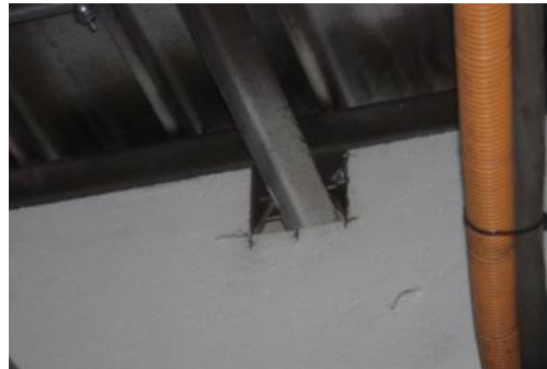
Figure 30: Structural members passing through a wall present a potential path of migration. Photo courtesy of Gladstein, Neandross & Associates, NREL
